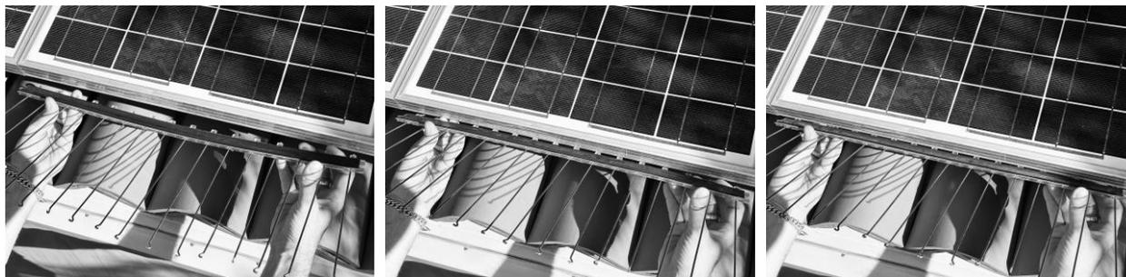
**N.B.!** At this stage, be careful to keep the adhesive tape or silicone spaced from the frame of the photovoltaic panel to avoid the "detach-attach" effect that would damage the effectiveness of the adhesive.
