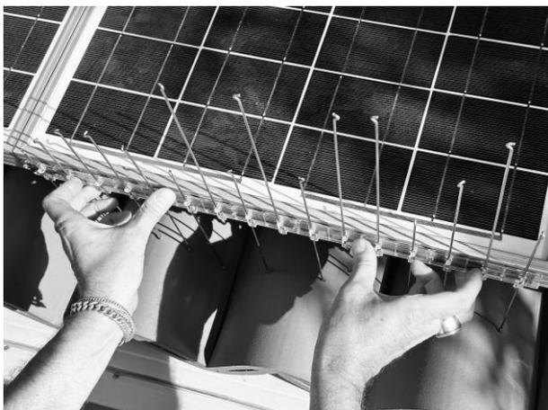
**3.7.6** Repeatedly press the entire length of the barrier with your fingers and/or the palm of your hands to obtain perfect adhesion of the barrier to the frame of the photovoltaic panel.
